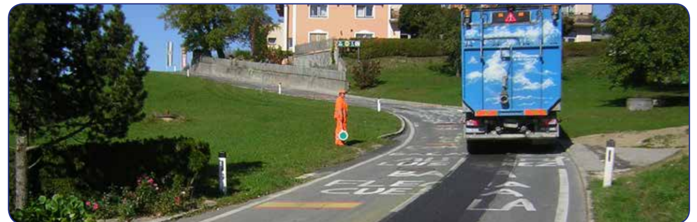
Removal of paint residues on a tarmac road after the World Cycling Championship
