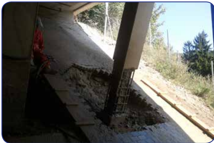
Concrete removal from bridge pillars by hand lances
