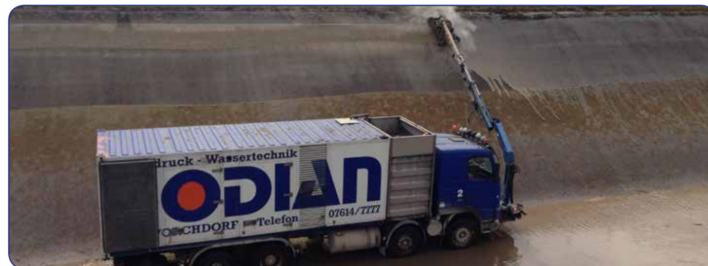
Surface preparation of power plant channel for renovation
