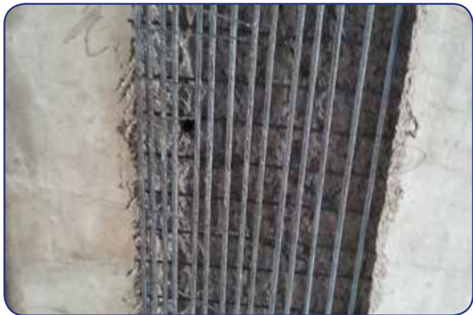
Concrete removal from the soffit
