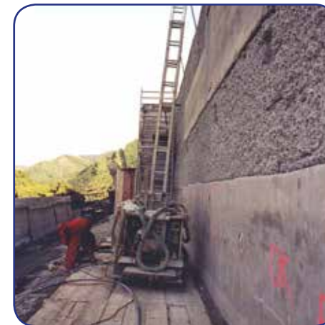
Concrete removal on vertical surfaces such as retaining walls, pillars, walls
