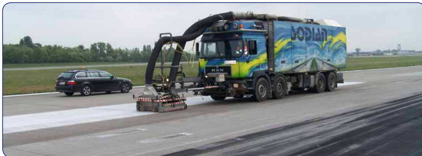
Removing rubber skid marks from tarmac and concrete pavement
