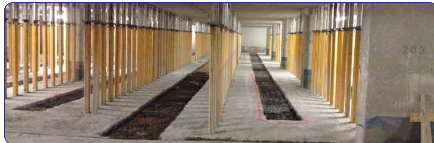
Concrete removal in an underground car park
