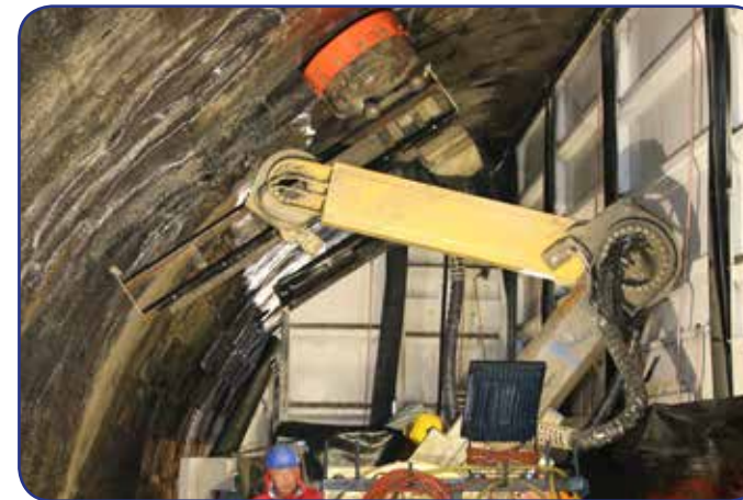
Stripping a rail tunnel without interrupting traffic
