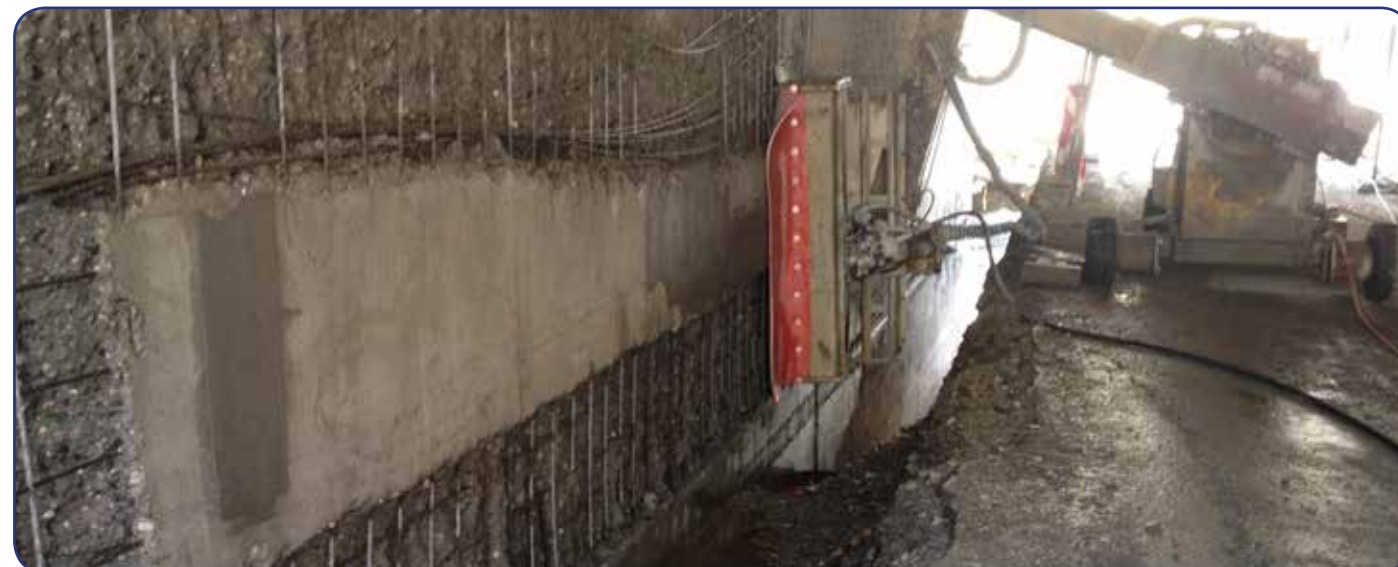
Concrete removal by pilgrim-step method
