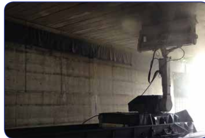
Soffit removal by robots from a wagon
