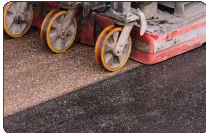
Removing rubber skid marks from tarmac and concrete pavement
