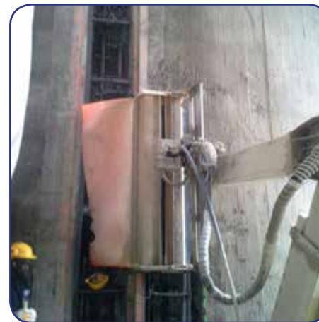
Concrete removal on vertical surfaces such as retaining walls, pillars, walls
