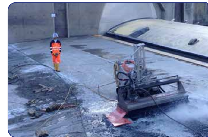
Concrete removal by robot
