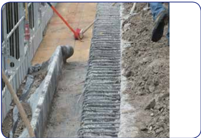
Cantilever after concrete removal
